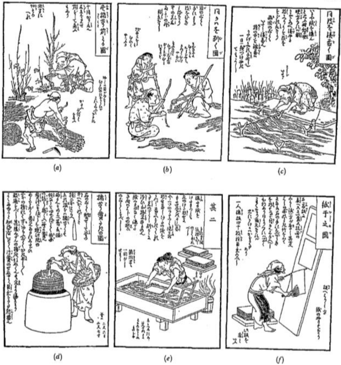
Appendix 106. 流漉 papermaking method in Japan, from the 紙漉重寶記, printed in 1798. Retrieved from Tsien (1985).
